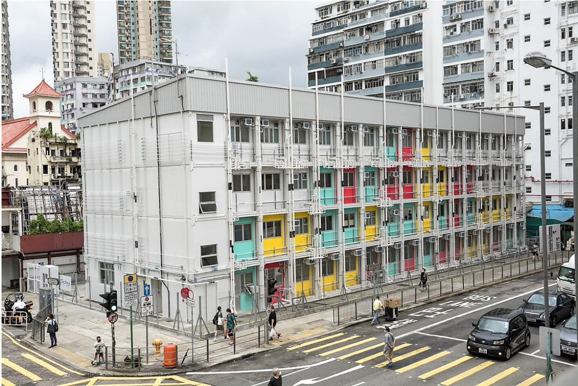
Figure 4: Nam Cheong Street Modular Social Housing Project (“Nam Cheong 220”), Sham Shui Po. Source: CIC MiC, https://mic.cic.hk/en/ProjectsInHongKong/3
